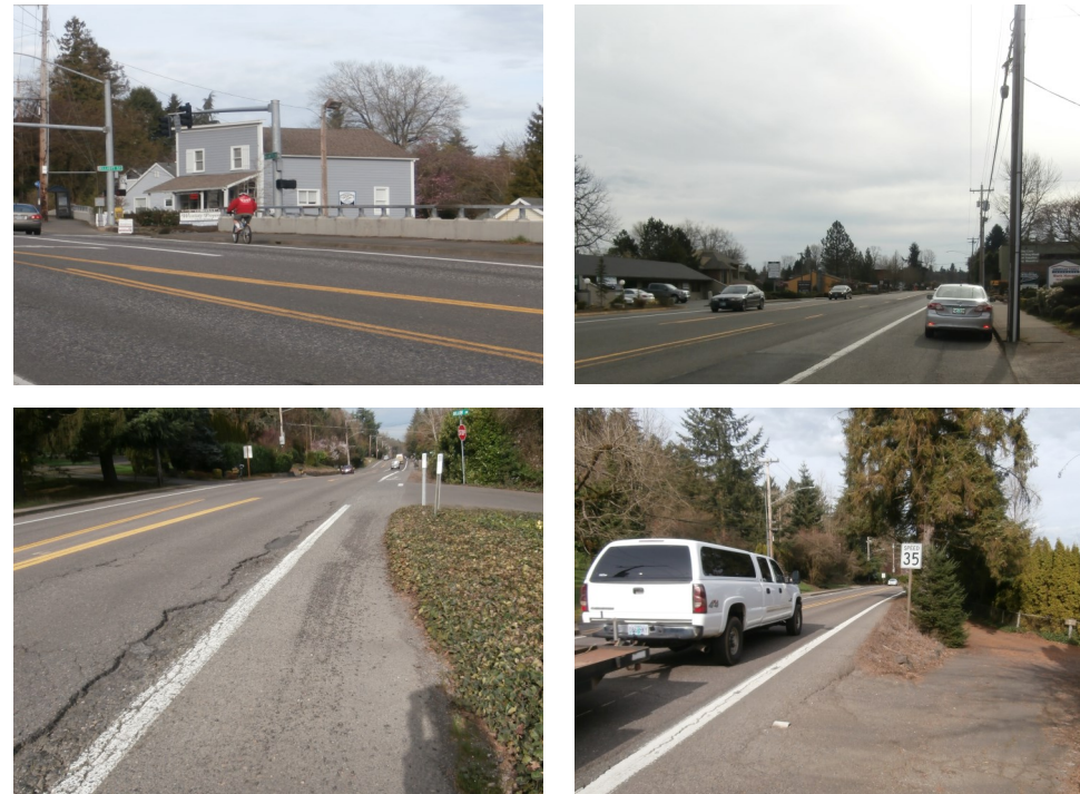
Existing bike facilities along OR 43 require bicyclists to deal with obstructions, gravel, limited shoulder space, and motor vehicles parked within bike lanes
