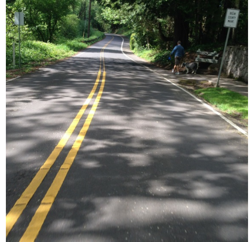
Photo 8: Old River Rd, potential alternate route
