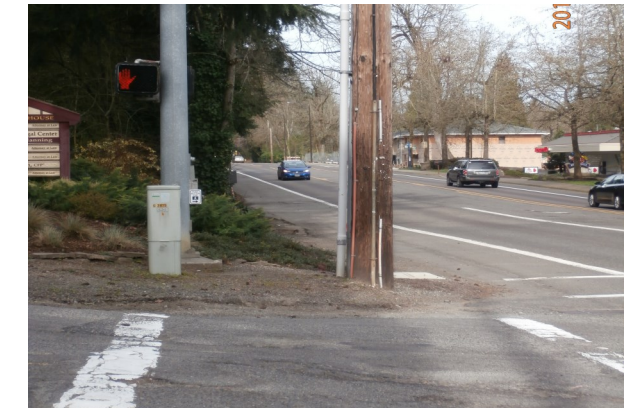
Marylhurst Drive at OR 43 traffic signal has no ADA accessibility at crossing and no sidewalks
