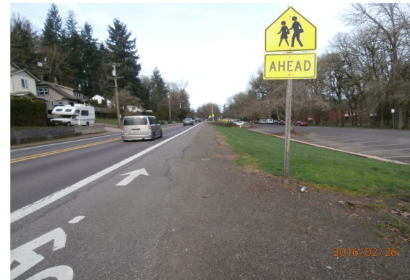
No sidewalk in front of Hammerle Park and substandard bike lane widths
