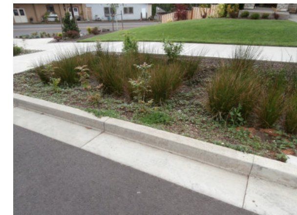
Example of rain garden Stormwater facility
