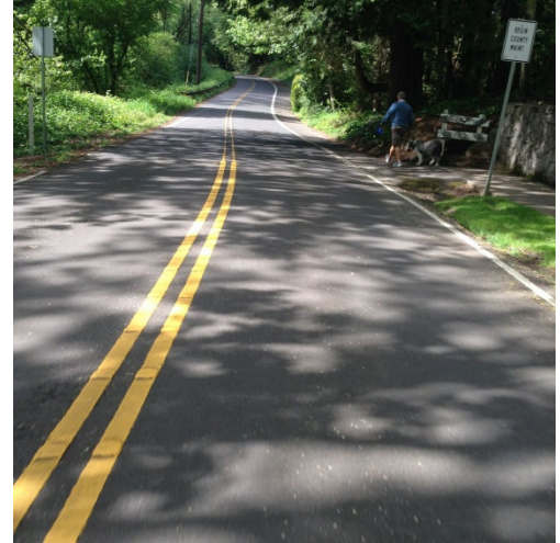
Photo 8: Old River Rd, potential alternate route
