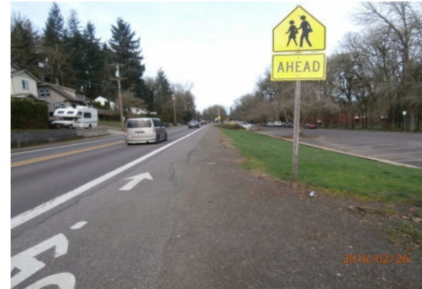
No sidewalk in front of Hammerle Park and substandard bike lane widths
