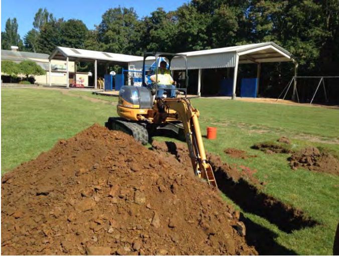
Photograph 1: Excavation of test pit TP-1 in progress.
