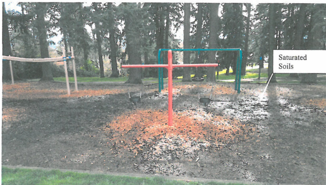
Photo 5. View of saturated soils more visible in the playground area. The Douglas fir trees below the playground have buttressed roots.
