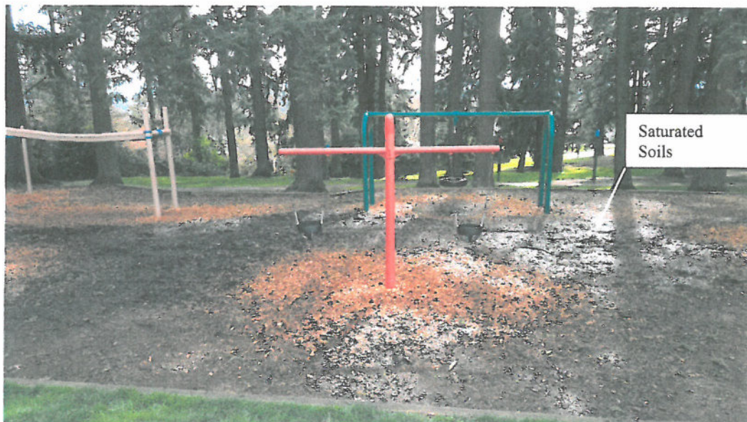
Photo 5. View of saturated soils more visible in the playground area. The Douglas fir trees below the playground have buttressed roots.
