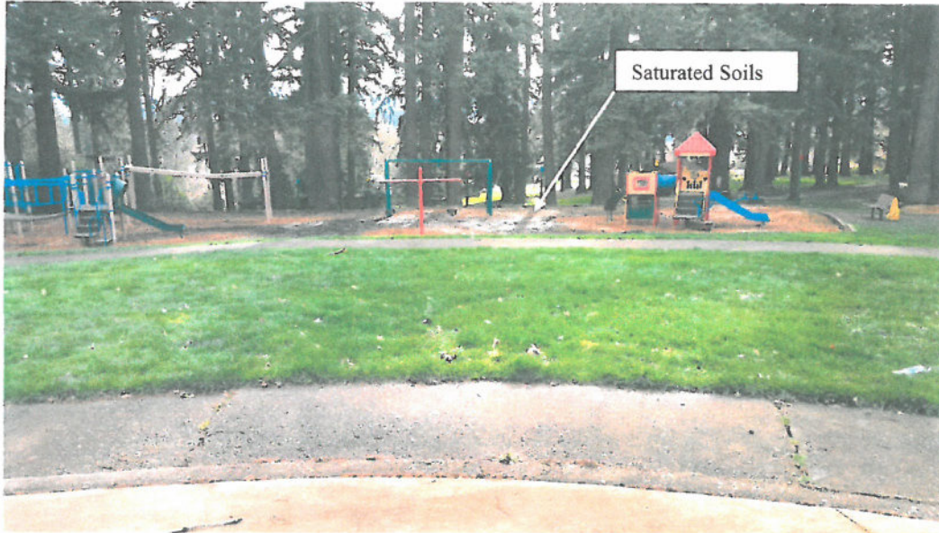
Photo 4. View looking south from the former wading pool towards the playground. The areas of saturated soils can be seen more easily in the playground area where storm water will try to infiltrate.
