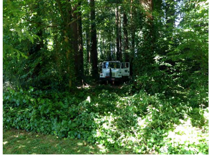
Photograph 2: Drill rig at boring B-3.
