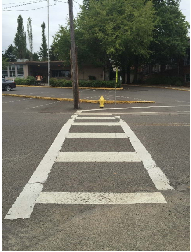
Exeter Crossing does not Connect Directly to the Building
