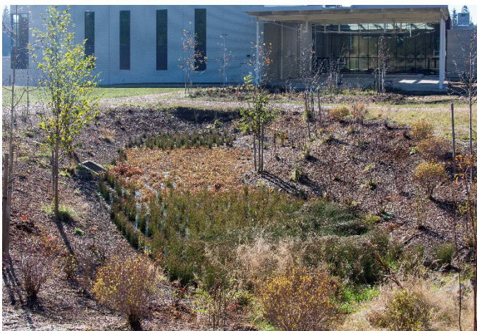
Figure 2: Stormwater Treatment & Detention Facility - Vernonia School
