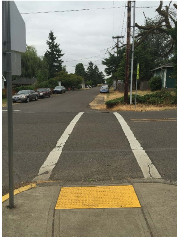
Sussex Crossing with No Sidewalks on South Side
