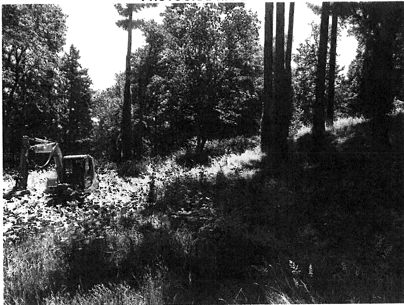
Subcontractor Excavating Test Pit TP-5, View to the South
