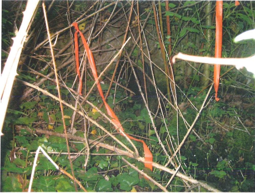
Photo Point 5 at entrance to culvert in nw corner of property
