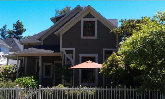
Compatible dormer addition that is on a side elevation, does not extend above the ridge of the roof, is minimally visible from the right-of-way, and has window opening proportions that are compatible with the existing residence.
