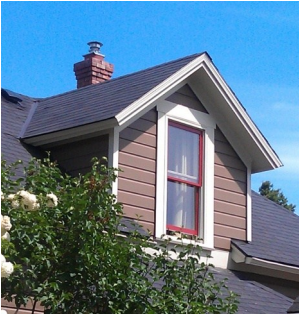
Compatible dormer addition that is on a side elevation, does not extend above the ridge of the roof, is minimally visible from the right-of-way, and has window opening proportions that are compatible with the existing residence.
