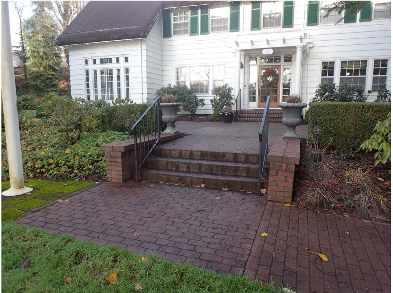
View: Looking north towards brick patio in front of façade.
