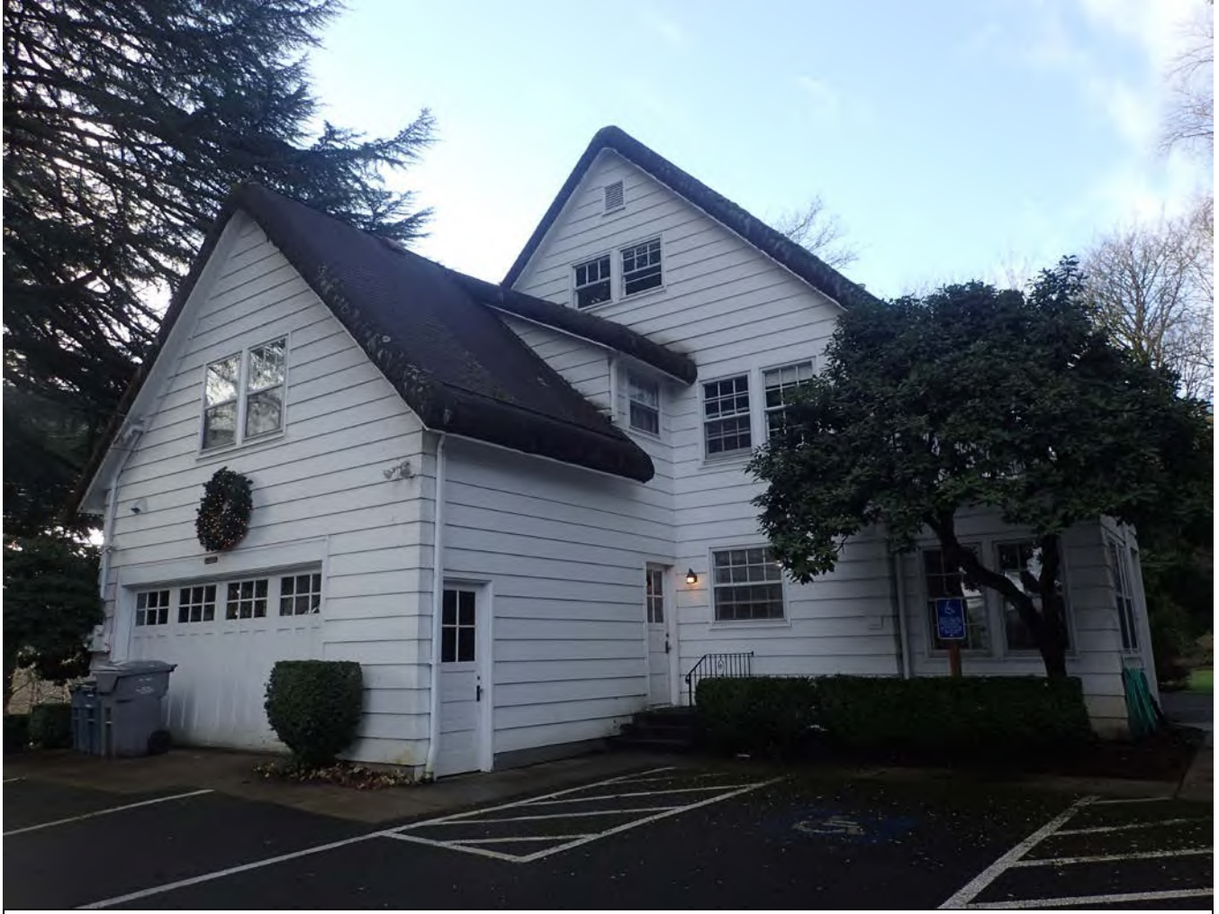
View: Looking south towards northeast elevation, including attached garage.
