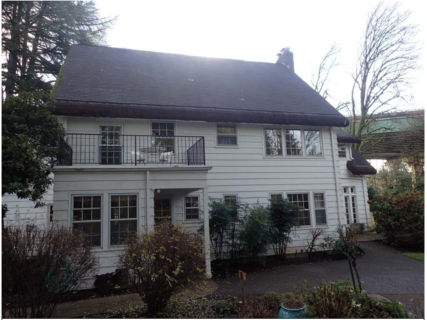
View: Looking southeast towards northwest (rear) elevation.
