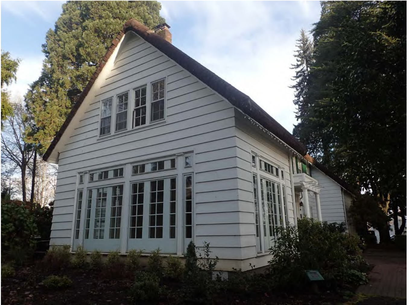
View: Looking northeast towards sunroom.
