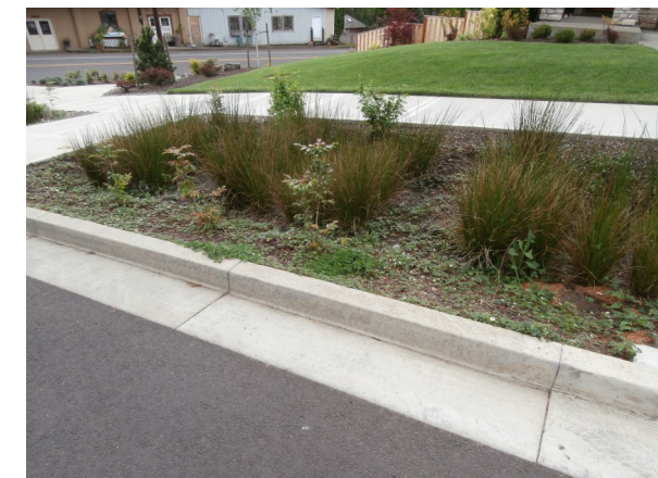
Example of rain garden Stormwater facility
