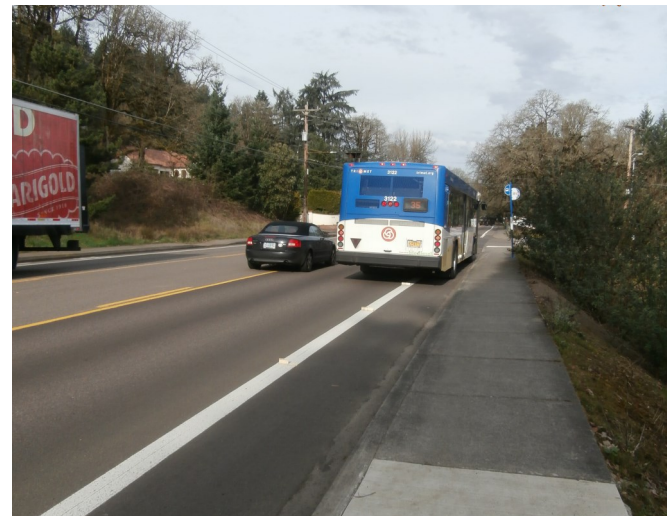
Many transit stops lack adequate shoulder space causing buses to block travel lanes
