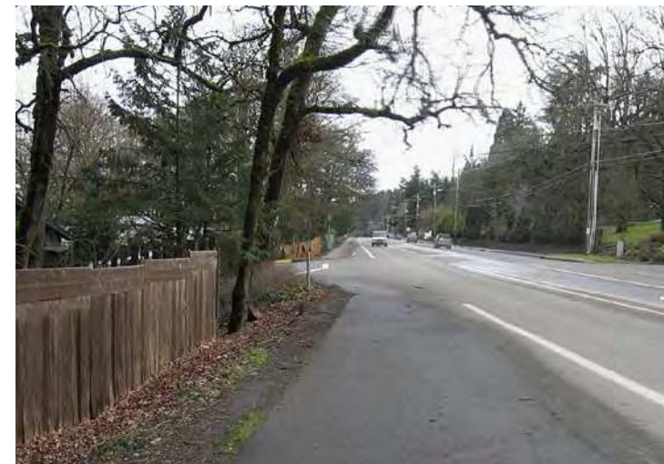
Existing conditions along OR 43
