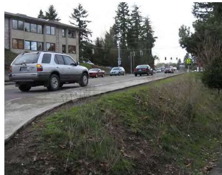
Steep slopes adjacent to and within the right-of-way sometimes limit the ability to expand existing facilities or provide new ones
