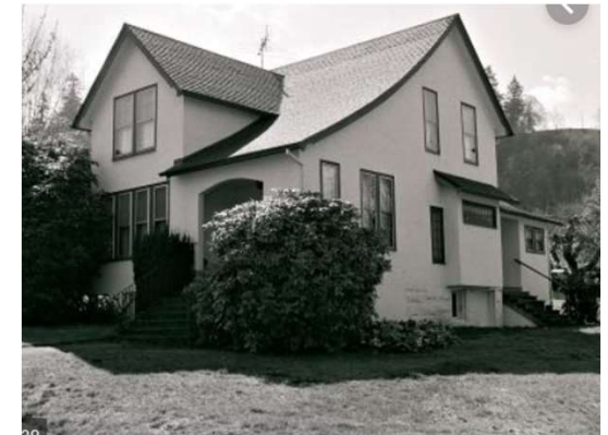
Cross-gable roof w/ Bellcast
