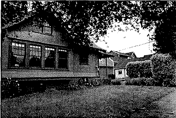
13 of 21: 13 th St, facing NW
