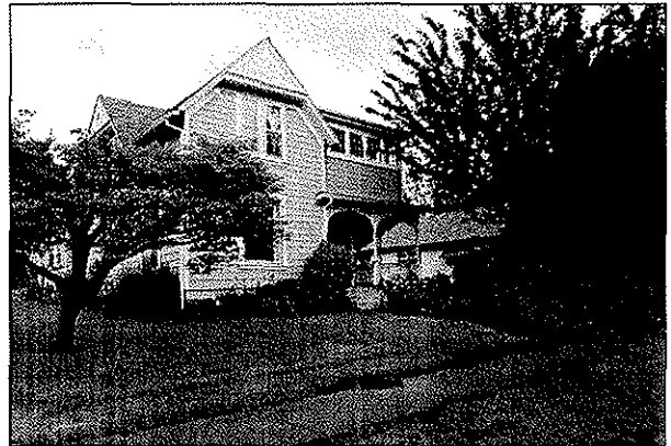
6 of 21: 4 th Ave, facing NE
