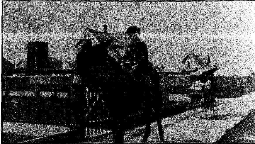
Figure 14: Corner of 6 th and 13 th , c. 1905 Note water tower in background.
