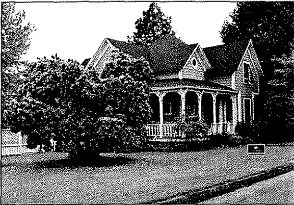
21 of 21: 5 th Ave. Facing SW
