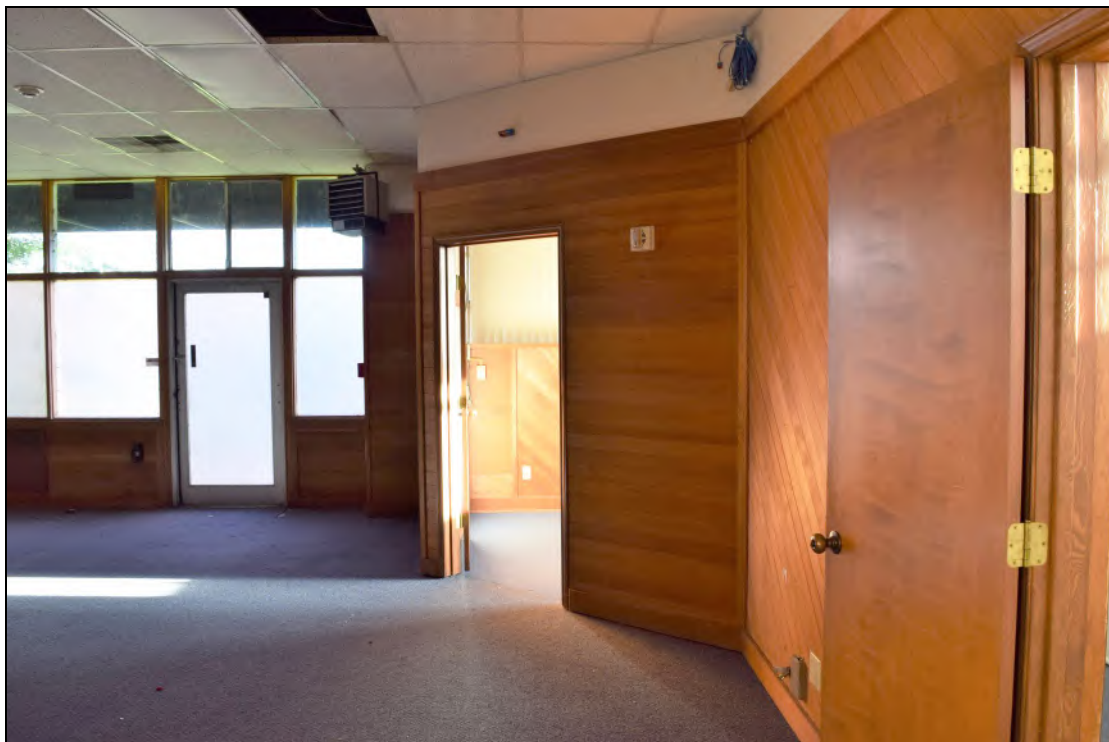
Photo 8 of 13: OR_Clackamas_HistoricCityHall_0008. Ground floor interior looking north at center front storefront bay (on left) and east-side offices (on right)
