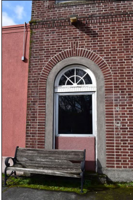
Photo 7 of 13: OR_Clackamas_HistoricCityHall_0007. Looking northwest at the original door opening leading upstairs (now a window) in the east wall.
