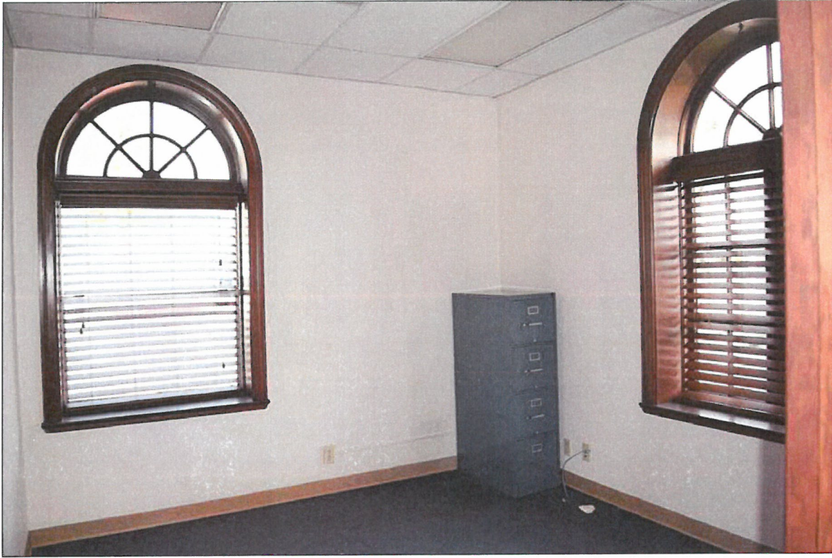
Photo 11 of 13: OR_Clackamas_HistoricCityHall_0011. Interior upper level looking north.
