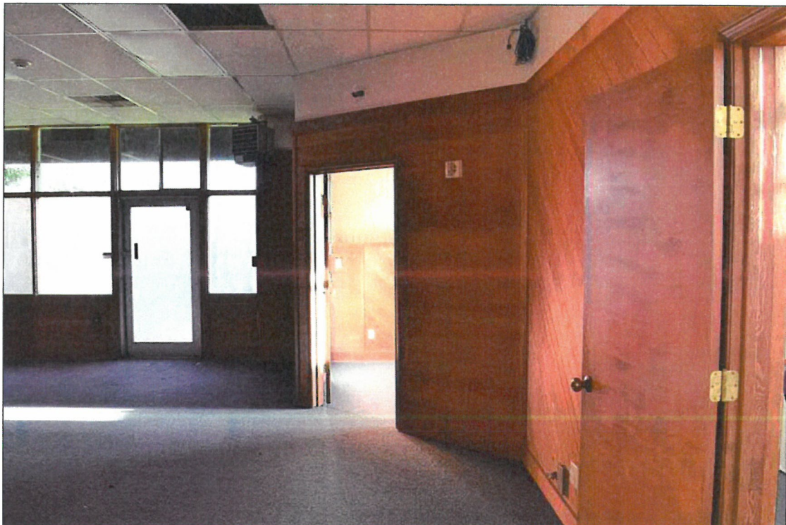
Photo 8 of 13: OR_Clackamas_HistoricCityHall_0008. Ground floor interior looking north at center front storefront bay (on left) and east-side offices (on right)
