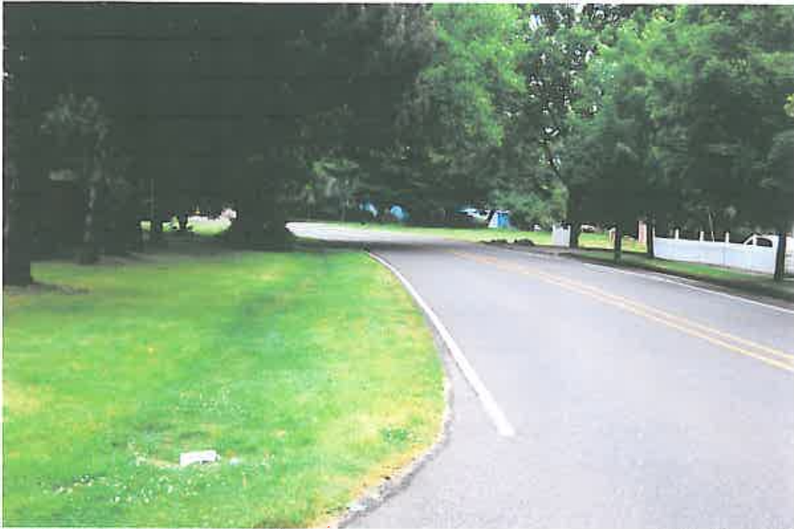
Photo 5 – Incomplete Projects - No sidewalks or bike paths on Will Falls Dr at 16 th St
