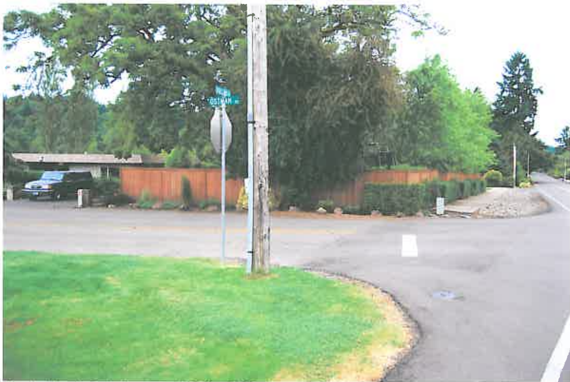
Photo 3 – Safety Issue at Dollar & Ostman – Sidewalk into utility pedestal & rocks.
