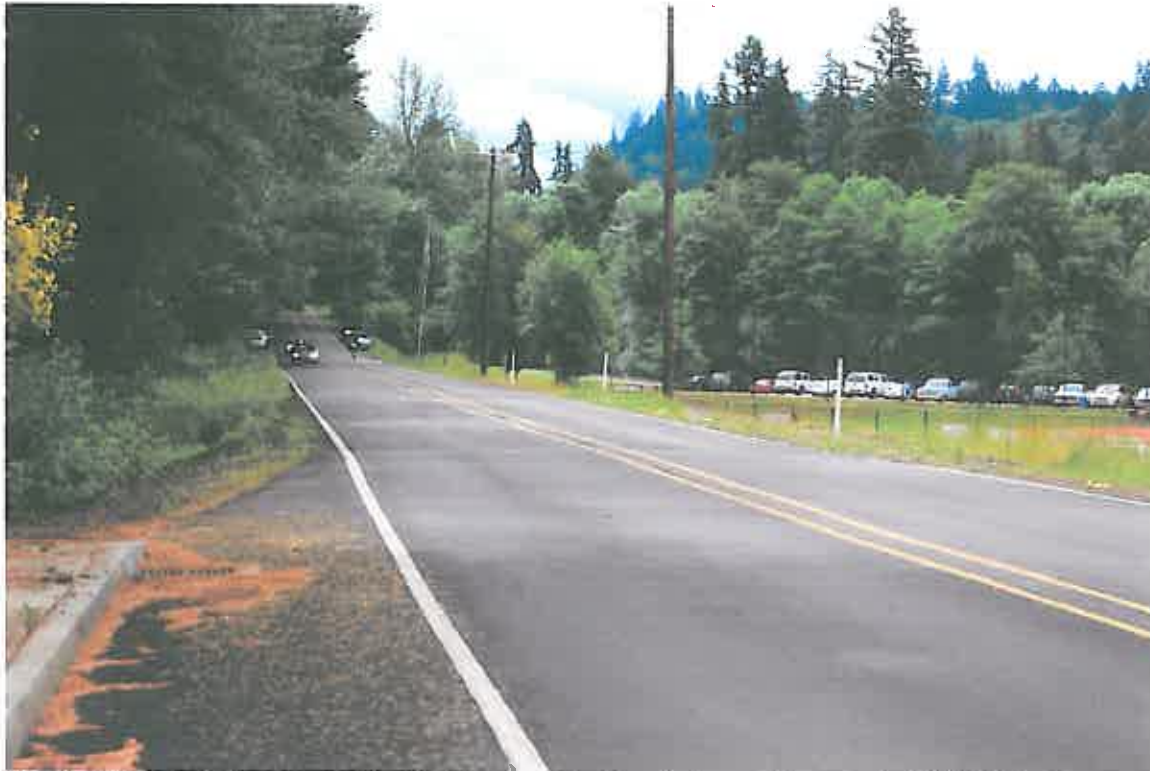
Photo 4- Safety Issue at Fields Park – Parking lot overflow onto Will Falls Dr, no bike path. There is summer weekly/monthly heavy park use during rush hour traffic.
