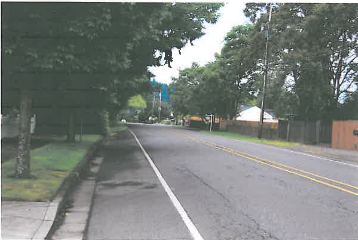
Photo 6 – Incomplete Projects - No sidewalks or bike paths on Will Falls Dr at 16 th St
