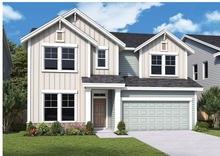
2124 Eleanor Road Detached Single Family City: West Linn State: OR Units: 1 Year Built: U/C (2025) Acres: 0.17 Du/acre: 6 Construction: Wood Frame Stories: 2
