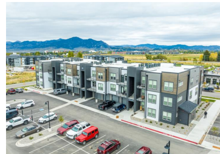
19 th and Graf Apartment Homes Low-Rise Garden Apartments City: Bozeman State: MT Units: 195 Year Built: 2023 Acres: 26.30 Du/acre: 7 Construction: Wood Frame Stories: 3
