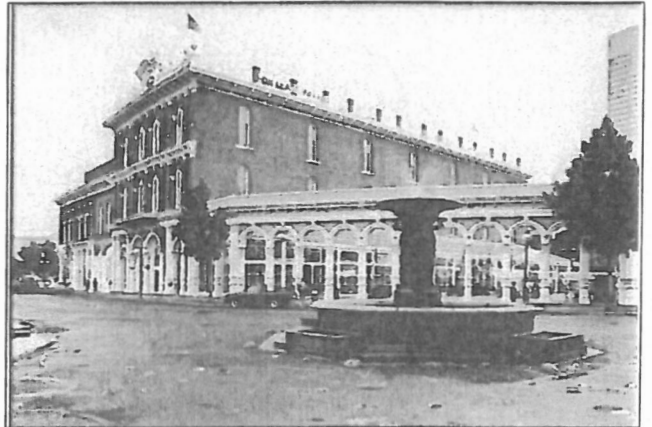
FIRST AVENUE - PORTLAND | CIRCA 1888 | CAST IRON COLUMNS
