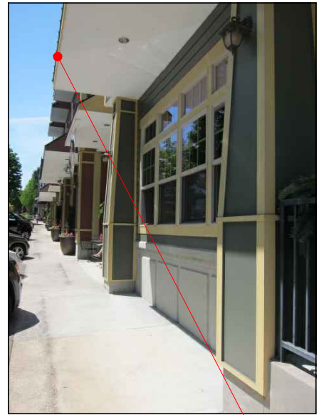
1980 WILLAMETTE FALLS DRIVE AWNING 24"+ FROM CURB
