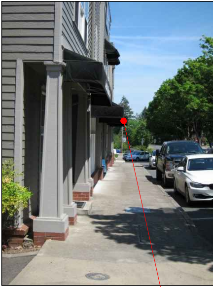
2008 WILLAMETTE FALLS DRIVE AWNING 48"+ FROM CURB
