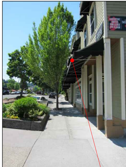
1880 WILLAMETTE FALLS DRIVE AWNING 36"+ FROM CURB
