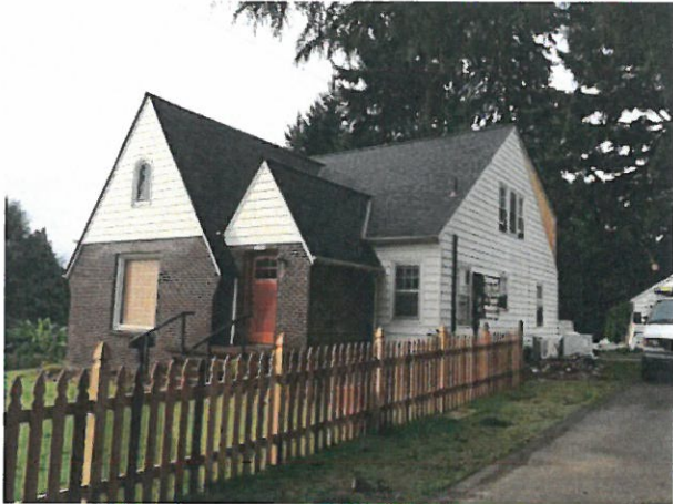
October 2013 – Front and side (north) elevation
