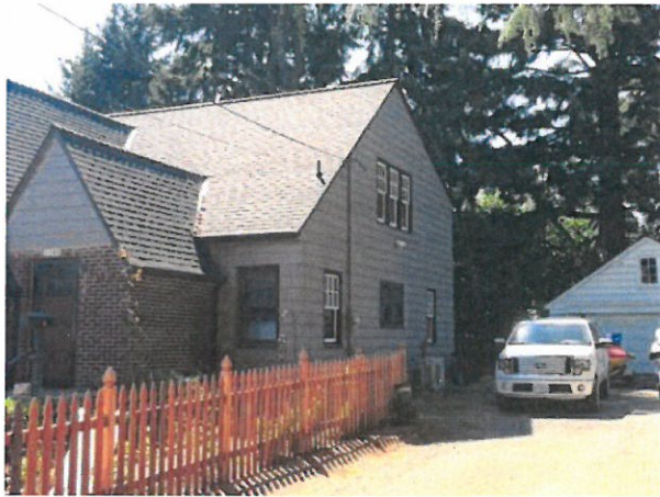
Side (north) Elevation – August 2014
