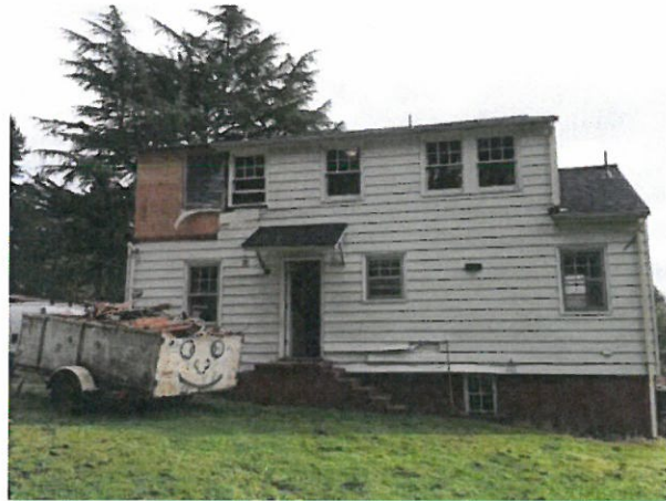
Rear elevation – October 2013
