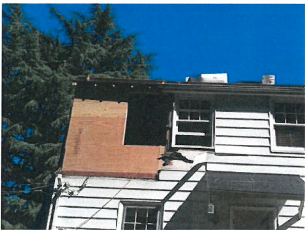
Rear elevation – September 2013
