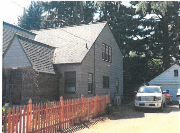
August 2014 – Side (north) elevation
