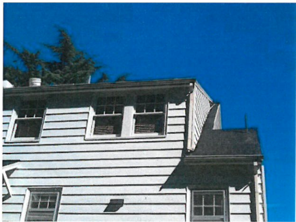
Rear elevation – September 2013
