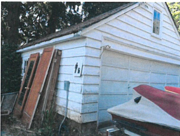
Existing garage – August 2014
