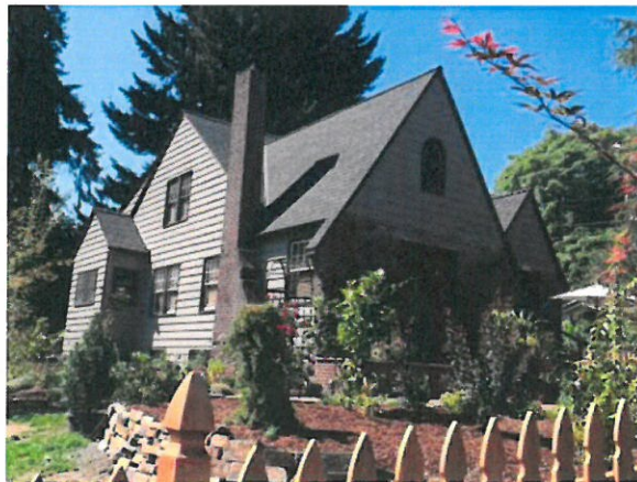
Side (south) elevation – August 2014
