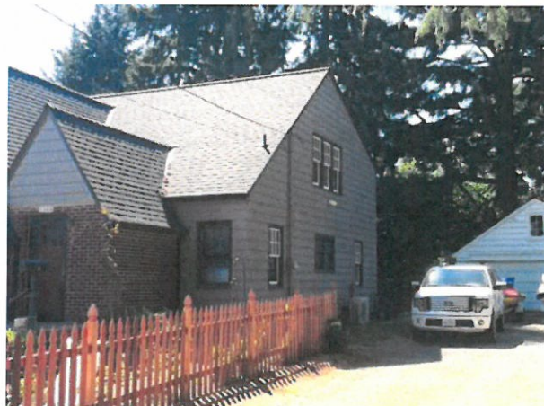
August 2014 – Side (north) elevation
