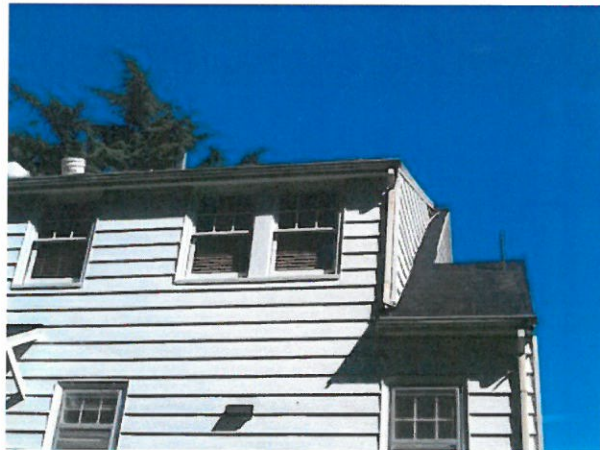
Rear elevation – September 2013
