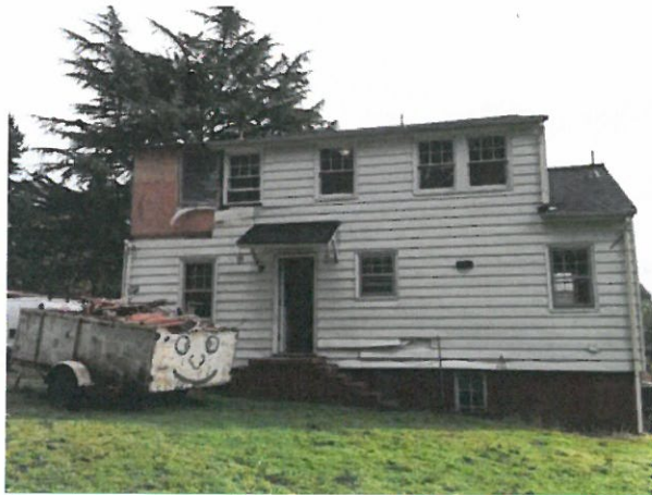
Rear elevation – October 2013
