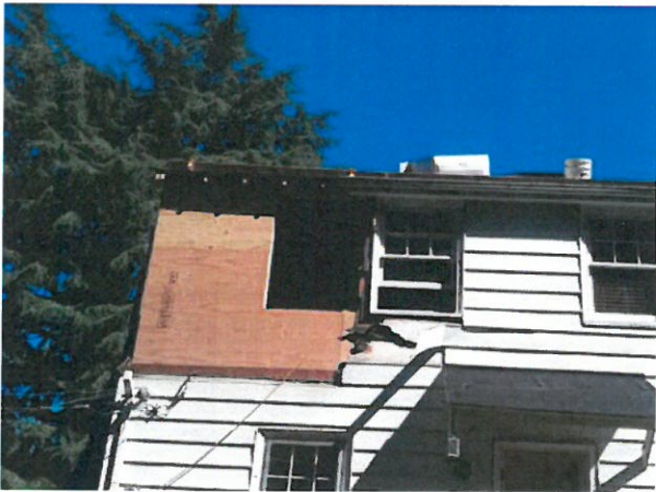
Rear elevation – September 2013
