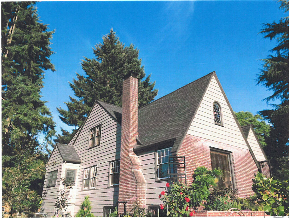
Photo of the house as it is currently, with restored original cedar siding and three-tab roofing.
