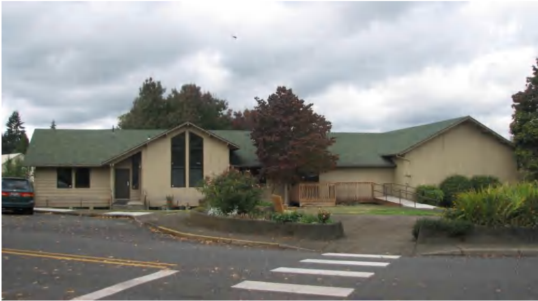
Front façade of building, set at angle facing 10 th Street/Willamette Falls Drive intersection. Although this is the visual front of the building, the site has an 8 th Avenue address. 8 th Avenue is north of the site, parallel to Willamette Falls Drive.
