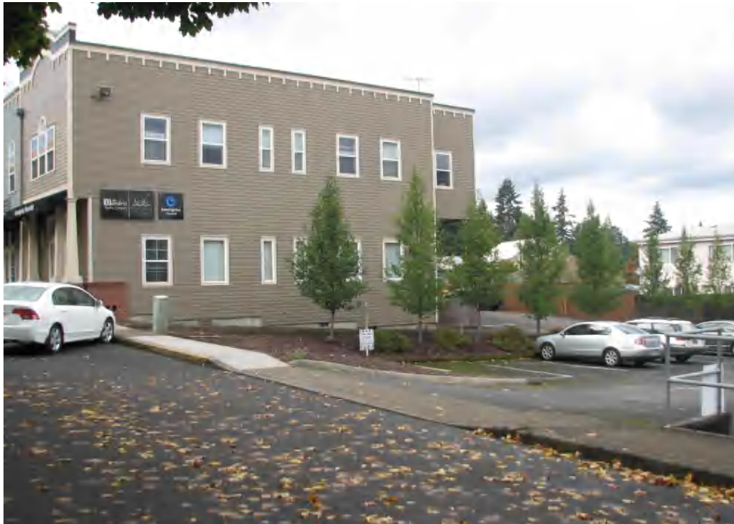
In the foreground above is the one vehicle ingress/egress to the site off of Willamette Falls Drive.
