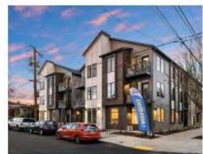
SE 11 th & Tenino Apartments Low-Rise Apartments
