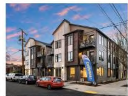
SE 11 th & Tenino Apartments Low-Rise Apartments
