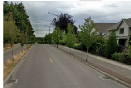
Separated Bike Facility
