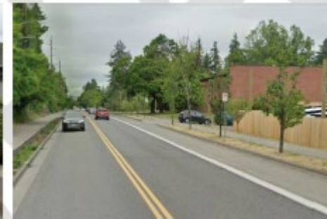
Separated Bike Facility
