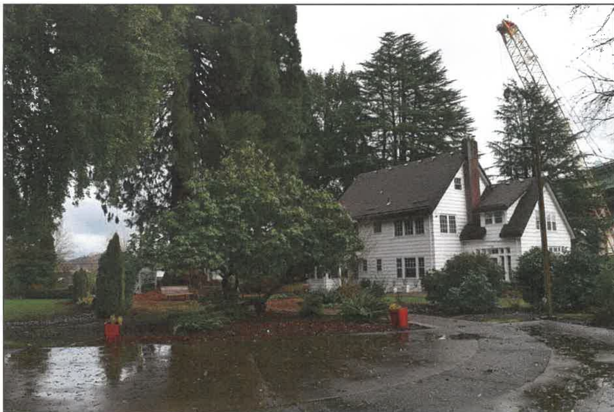
Photo 5 of 15: OR_ClackamasCounty_McLeanHouse_0005 Looking east at 'west' and 'south' walls of house and large trees nearby.
