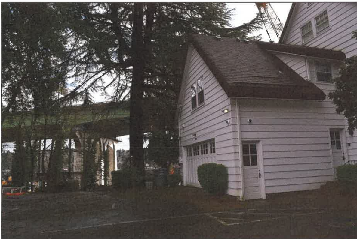
Photo 3 of 15: OR_ClackamasCounty_McLeanHouse_0003 Looking south at garage and kitchen doors.
