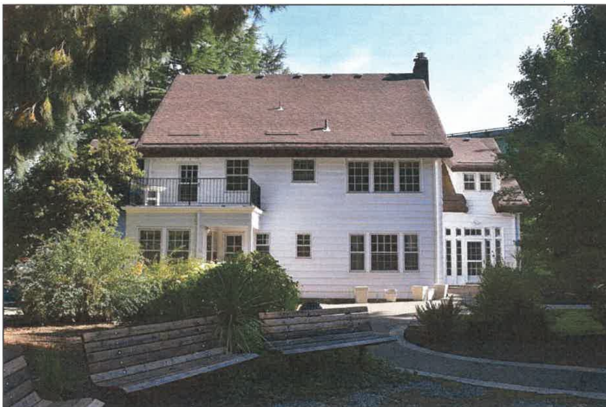
Photo 4 of 15: OR_ClackamasCounty_McLeanHouse_0004 Looking southeast at rear façade.
