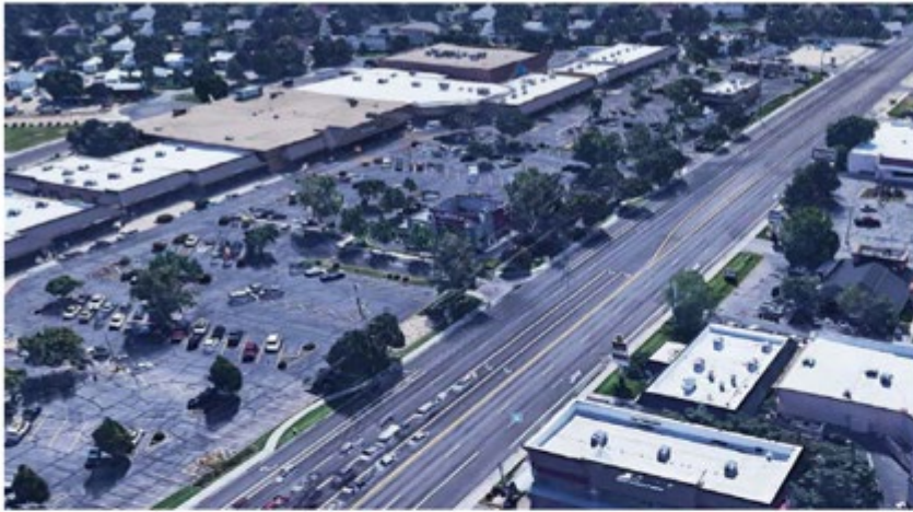
photos (top to bottom) Existing Glenwood station area. The concept developed builds off of the recent improvements to the business facades on the north side of State Street.
