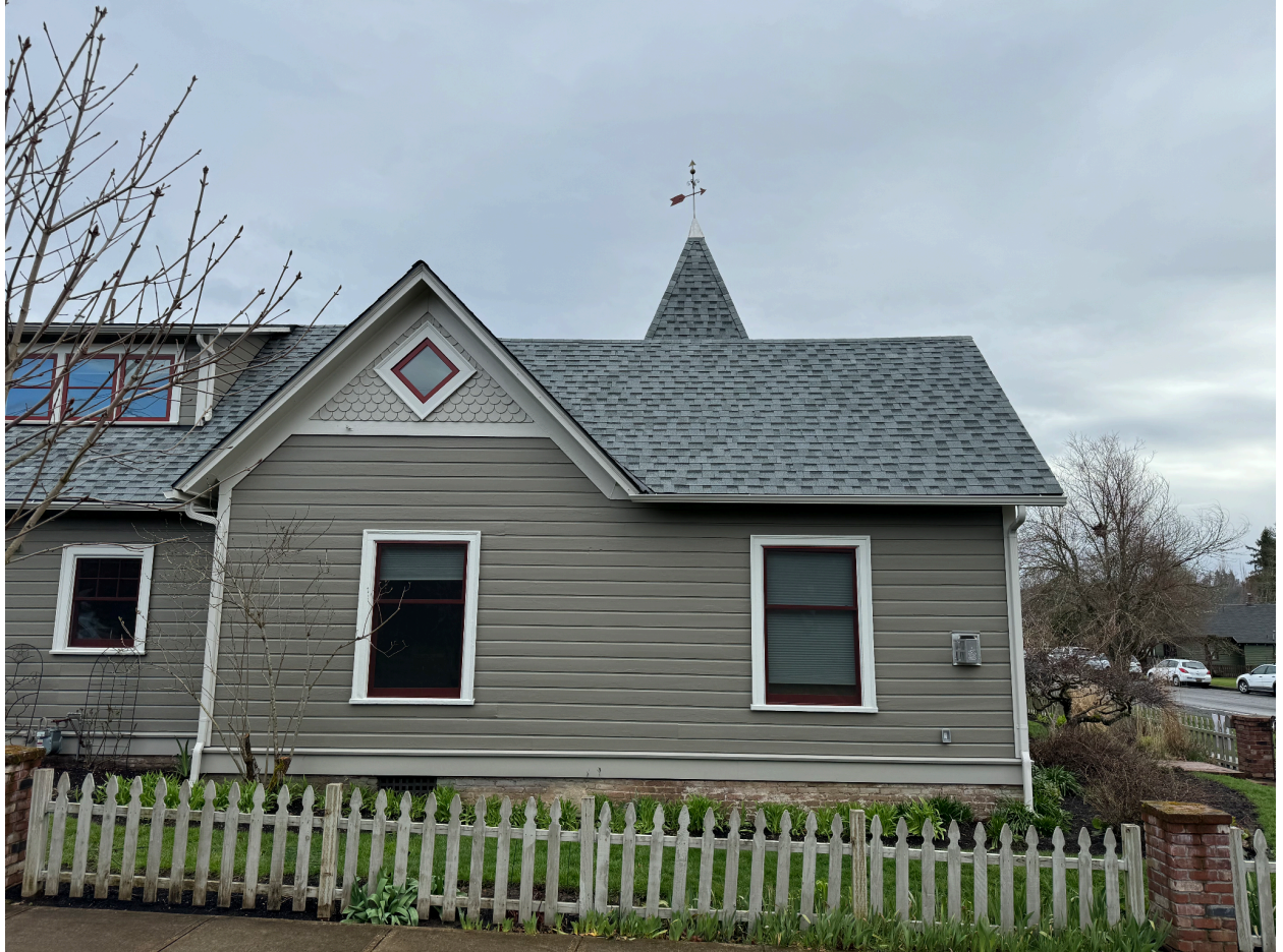
Photo of West Elevation - 13th Street 2024
