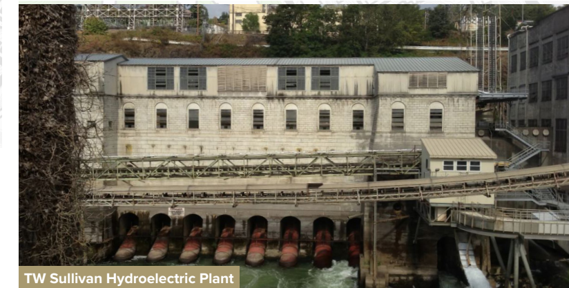
TW Sullivan Hydroelectric Plant
