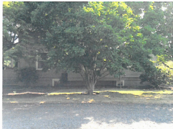
West (right) elevation of existing residence, the left window is proposed to be enlarged
