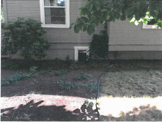
Existing basement window and well
