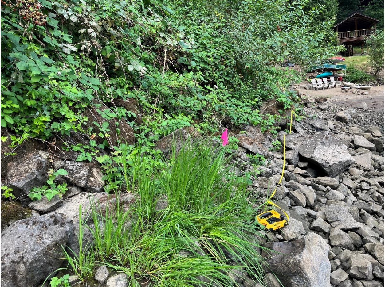
Figure 7b. Ground level photograph of DS-2a facing west.
