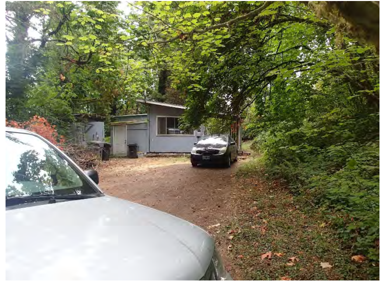
View facing east towards house from the gravel driveway.
