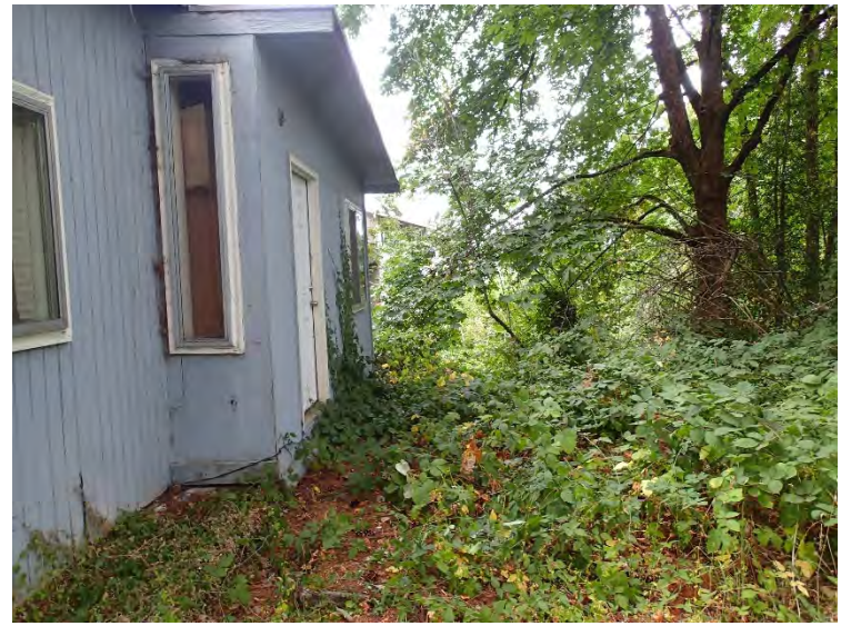
View on the east exterior of the house facing north.
