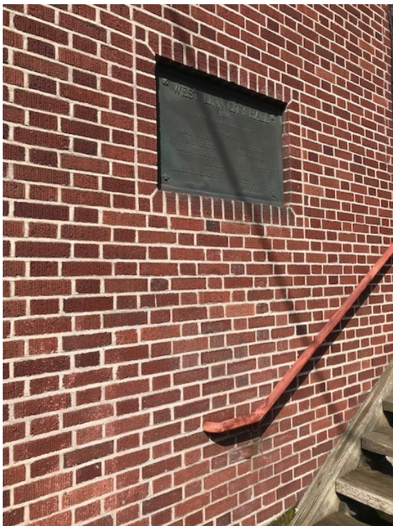
Front of Building
