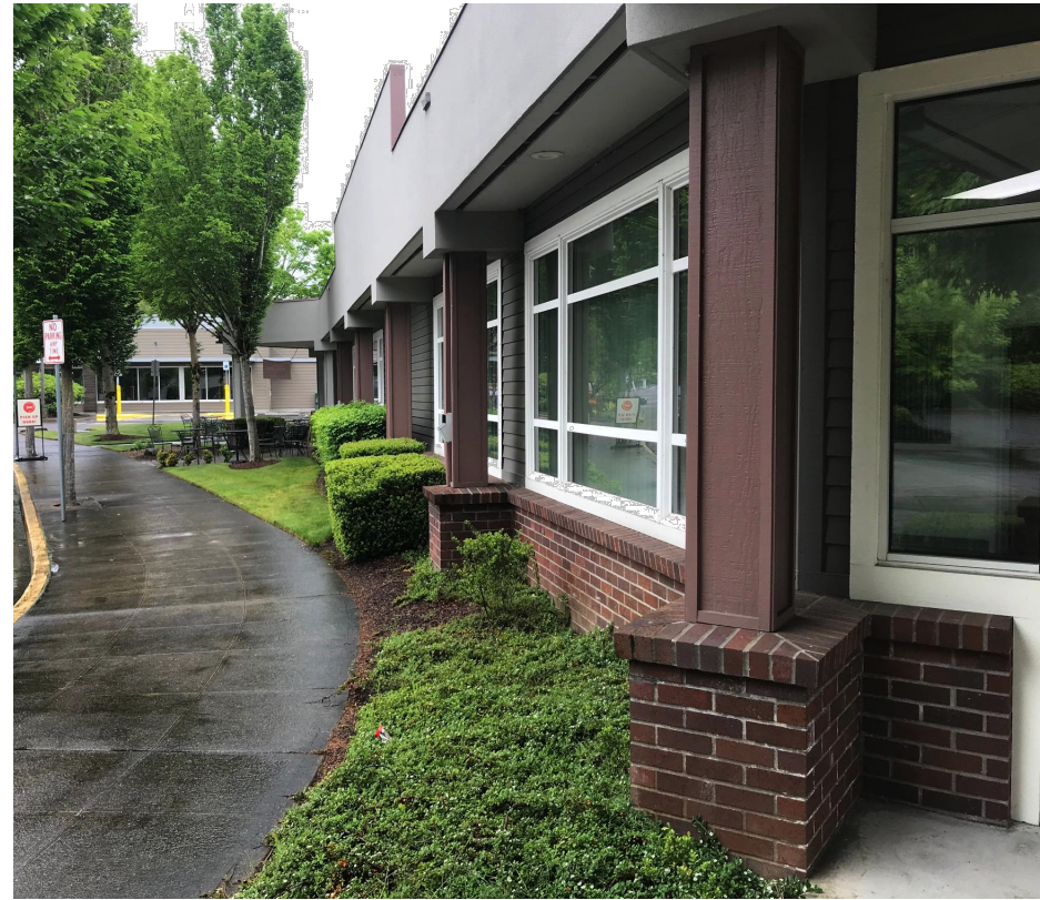
2 EXISTING SOUTH VIEW
