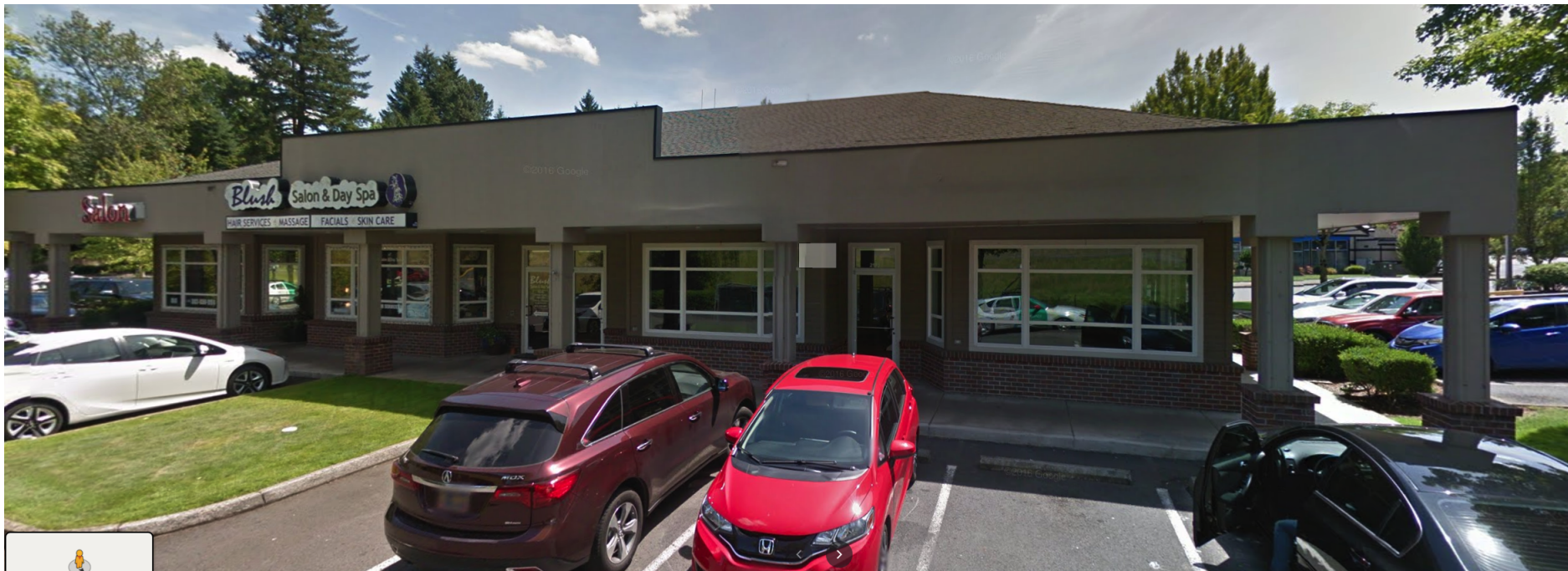
3 EXISTING NORTH VIEW
