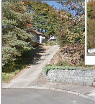
2463 Tipperary Court – 33% driveway grade
