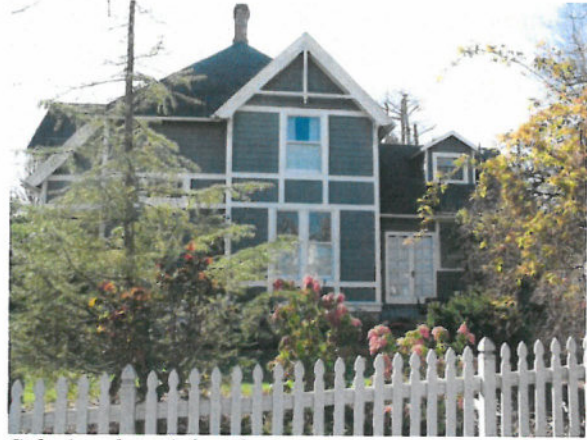
Side (northeast) façade
