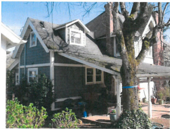
Rear (northwest) façade
