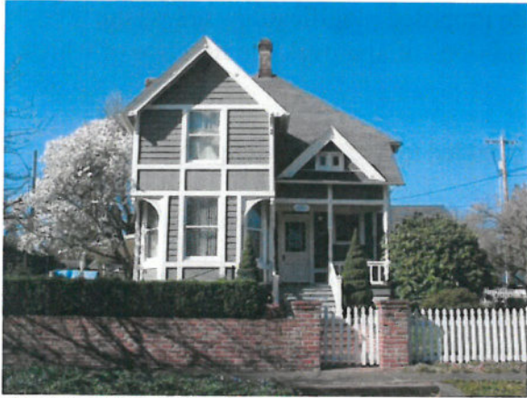
Front (southeast) façade
