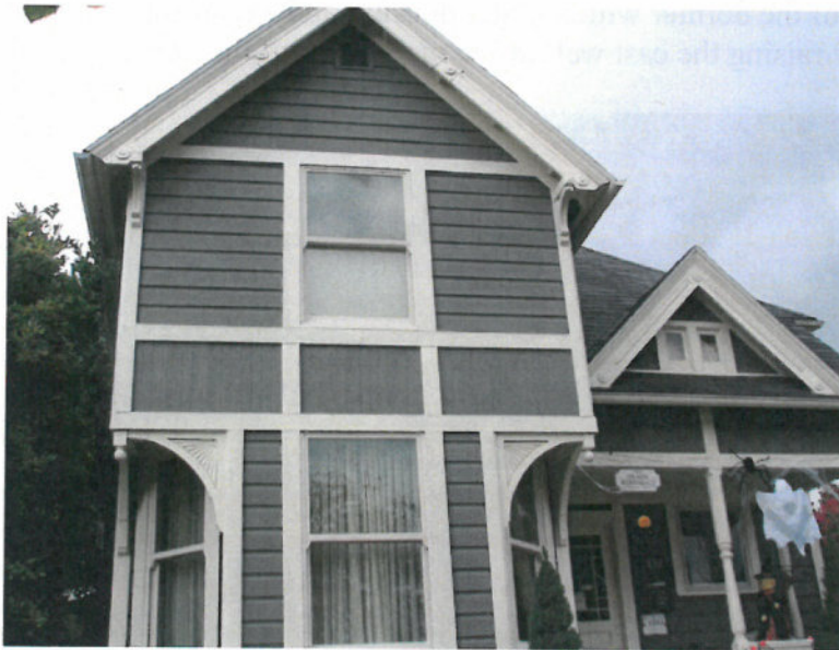
Front façade, will not change.
