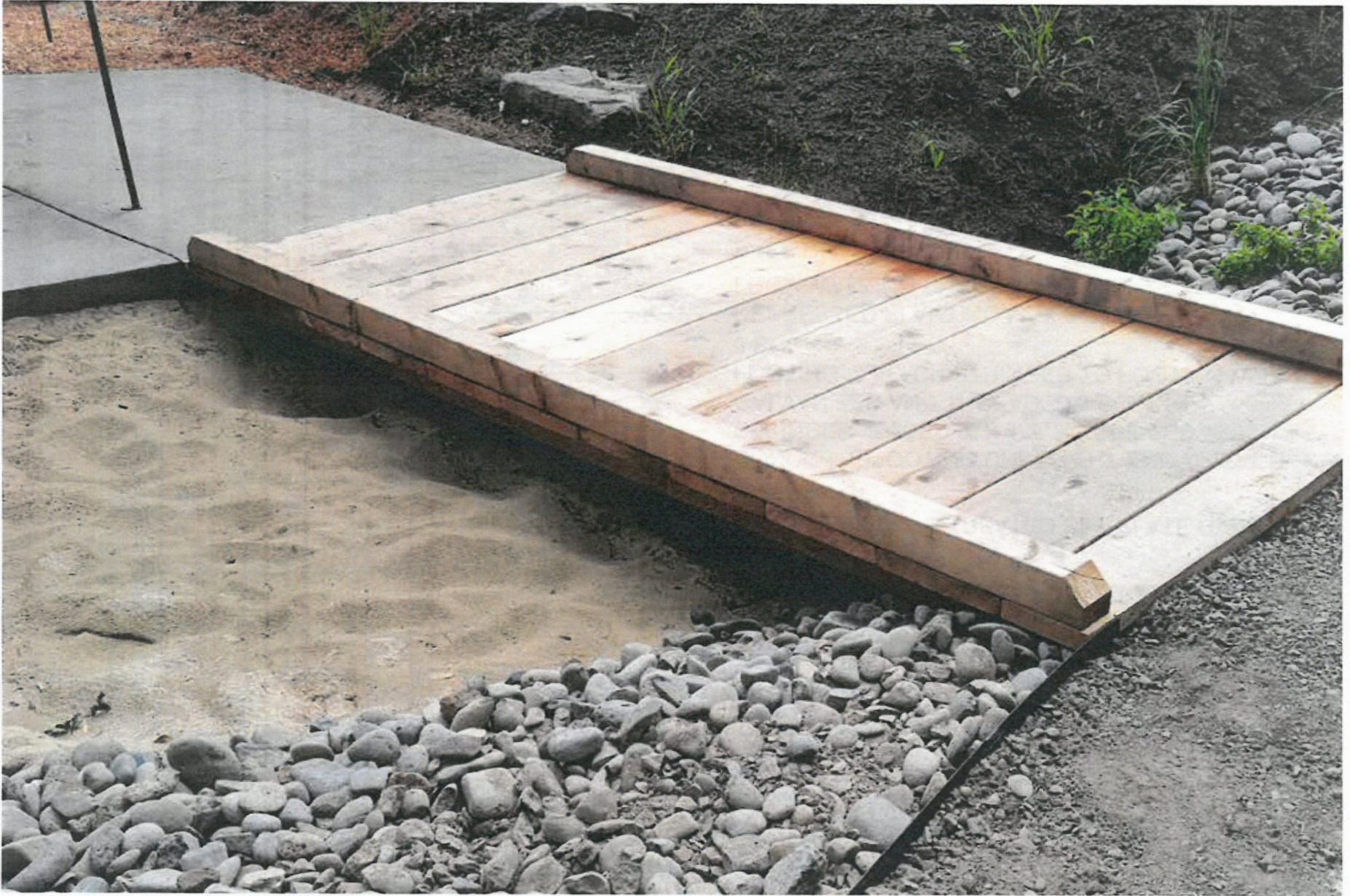
Foot Bridge - Example
