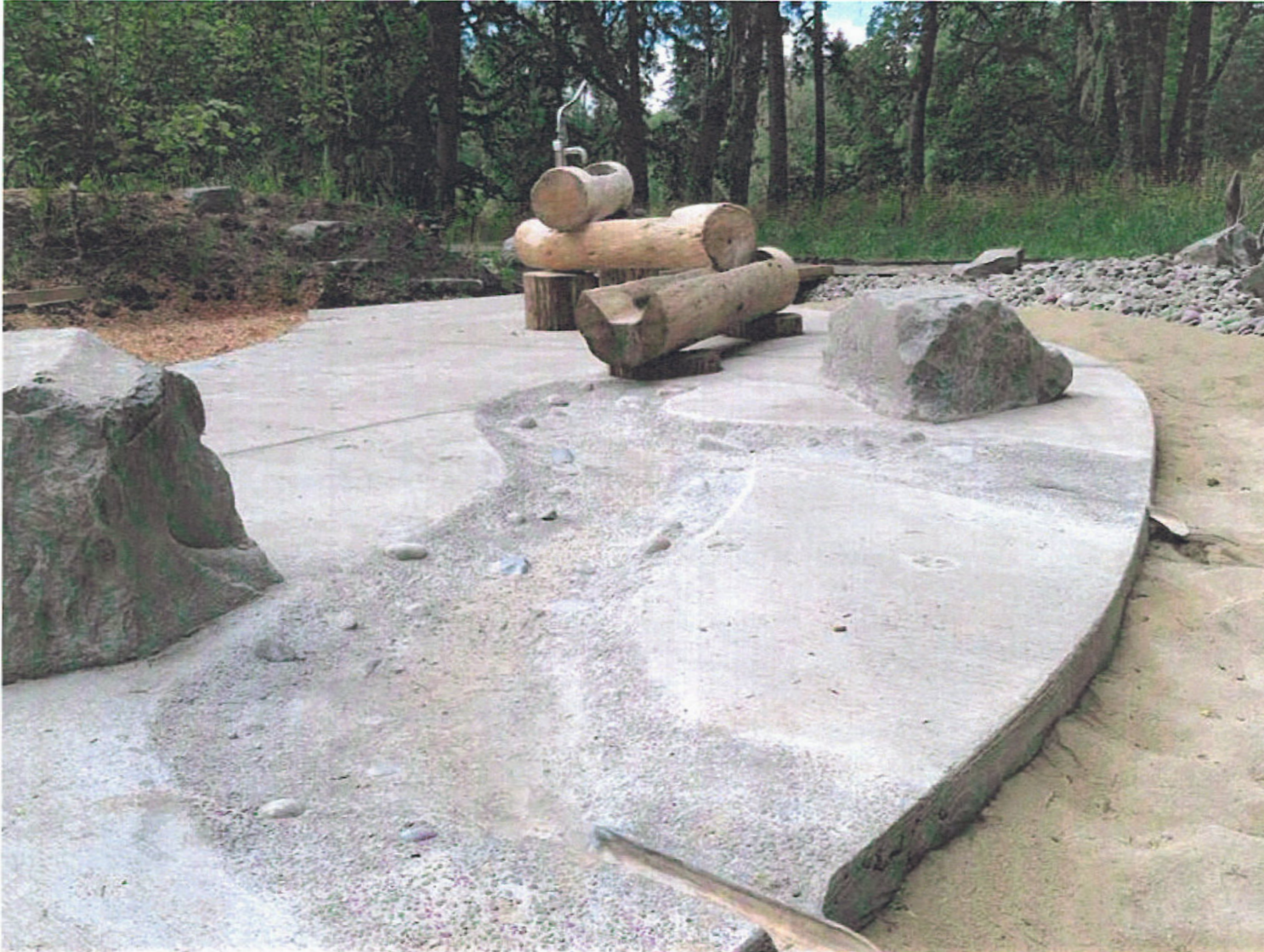
Concrete Water Course - Example
