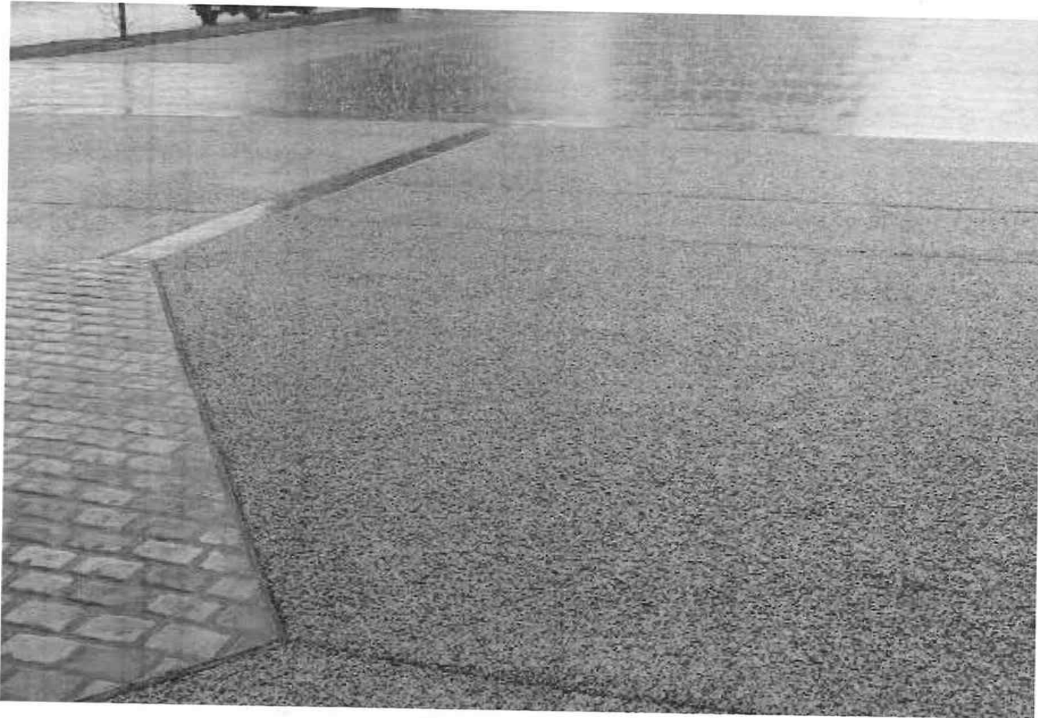
Porous Concrete Paving - Example
