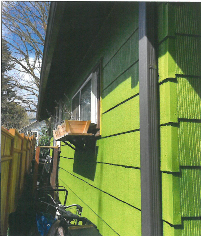
SIDE ELEVATION - WEST View Along West Fenceline
