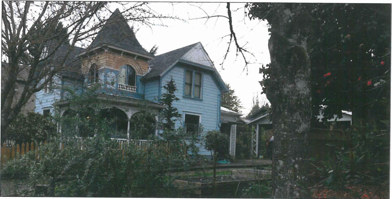
NEIGHBOR TO THE WEST AT 1724 4th AVENUE View From Sidewalk Looking Northwest
