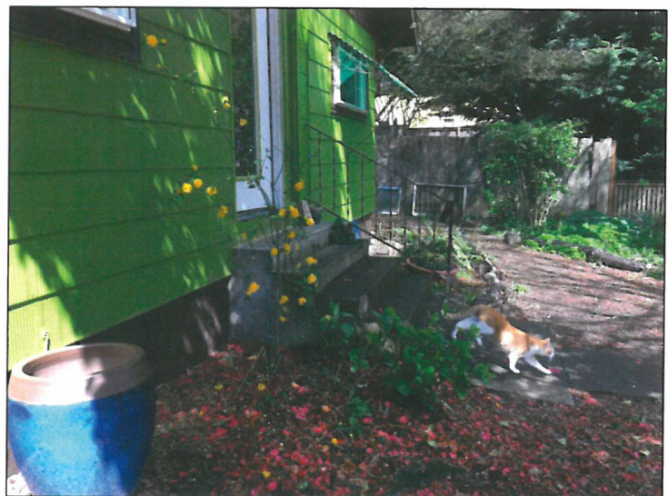
FRONT ELEVATION - SOUTH Detail of Concrete Steps
