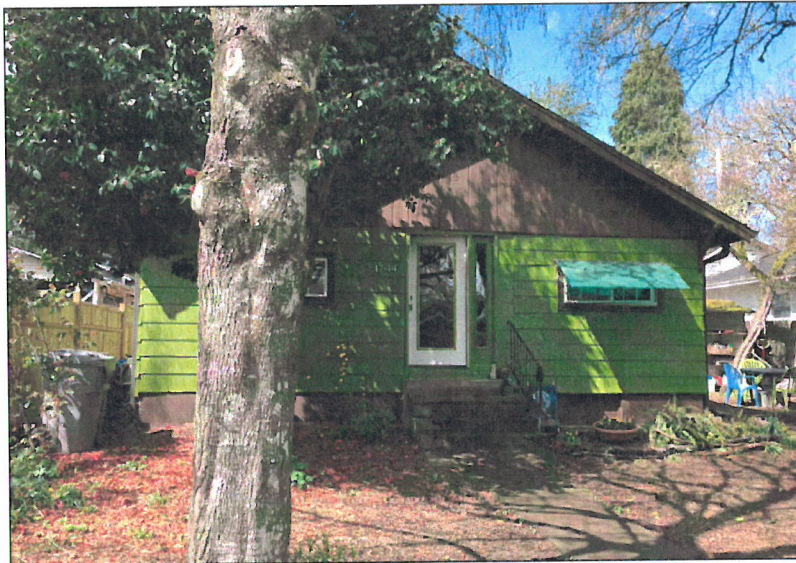
FRONT ELEVATION - SOUTH Street View From Sidewalk
