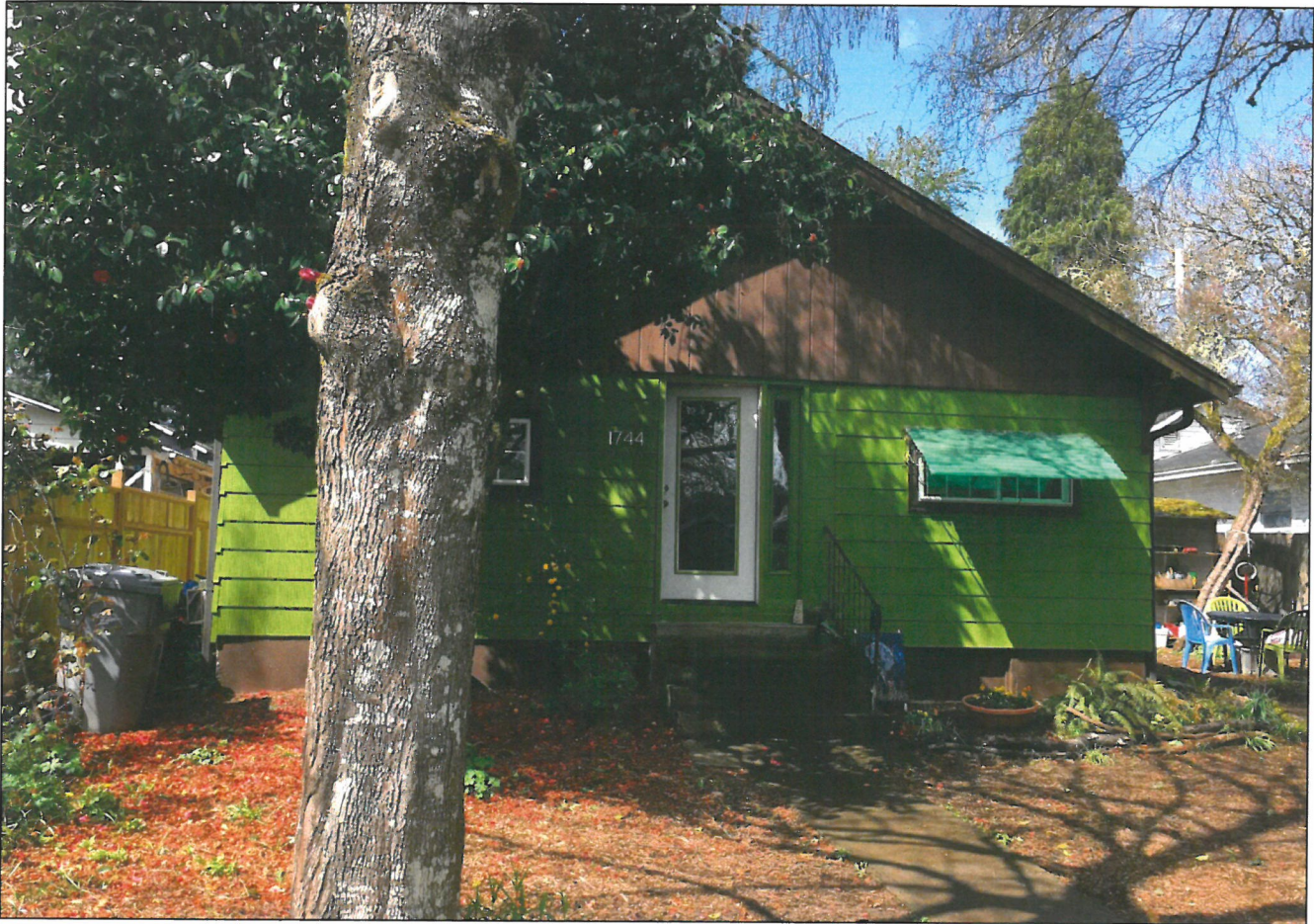
FRONT ELEVATION - SOUTH Street View From Sidewalk
