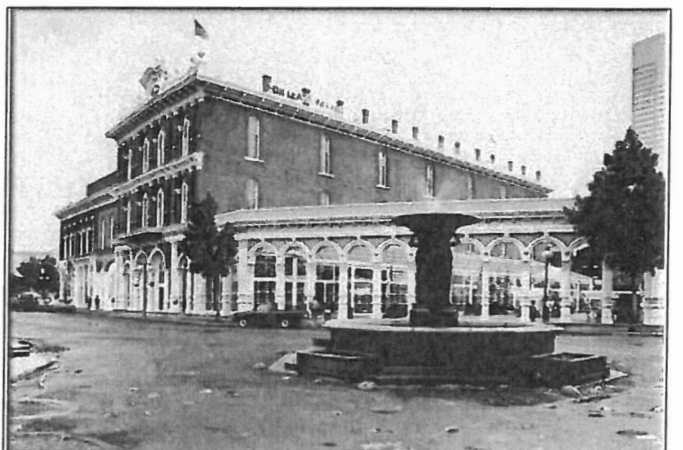
FIRST AVENUE - PORTLAND | CIRCA 1888 | CAST IRON COLUMNS
