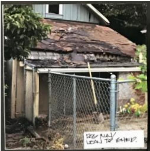
Noncontributing Accessory Structure Addition
