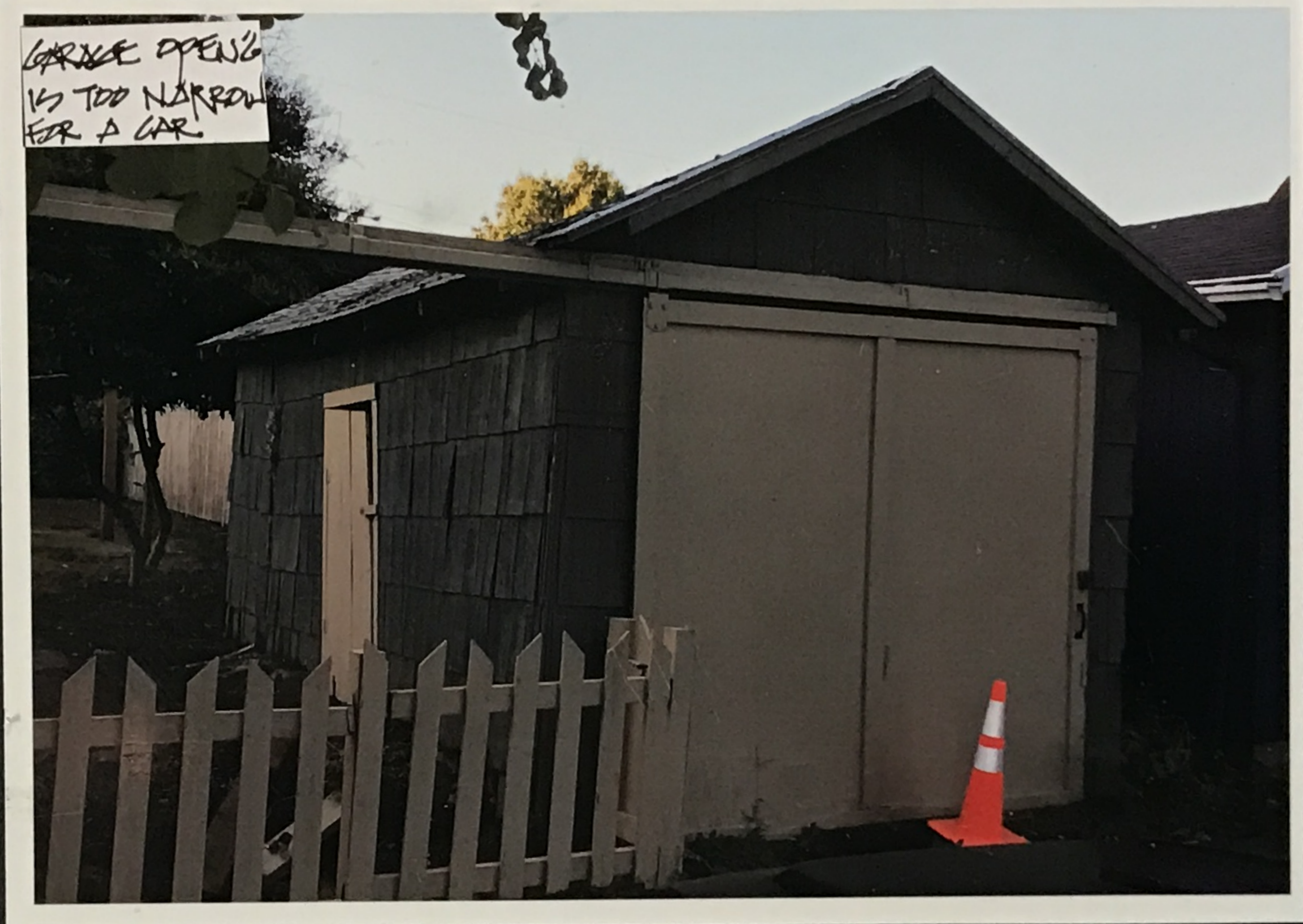
SEVERE BOW IN GARAGE RIDGELINE
