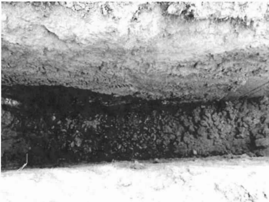
Test Pit TP-10
