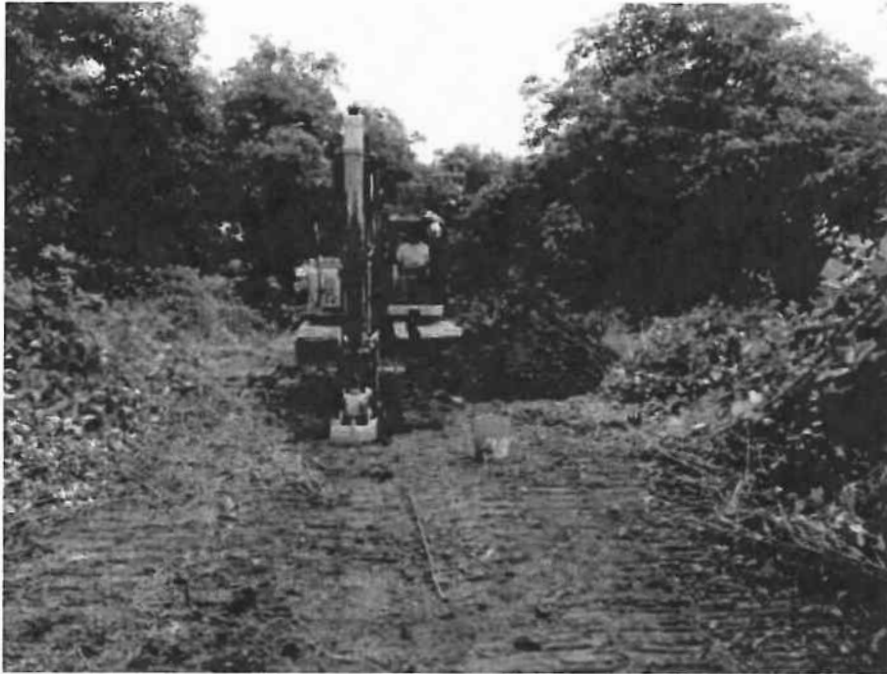
Test Pit TP-1
