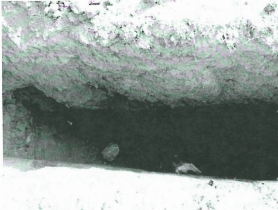
Test Pit TP-2
