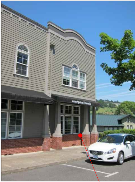
2008 WILLAMETTE FALLS DRIVE SILL @ 38" ABOVE SIDEWALK
