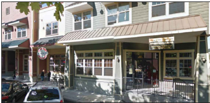
1980 WILLAMETTE FALLS DRIVE
