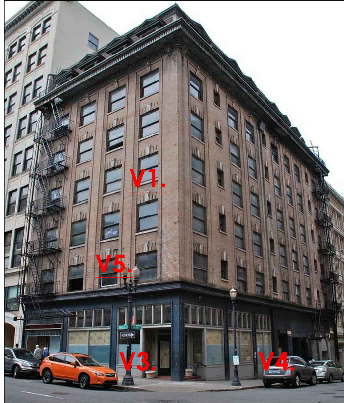
SW ALDER ST. & PARK AVE. - PORTLAND
