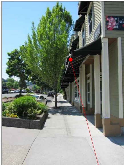
1880 WILLAMETTE FALLS DRIVE AWNING 36"+ FROM CURB
