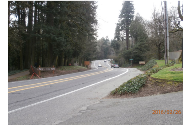
Mary S. Young Park along OR 43 lacks sidewalks on both sides of highway
