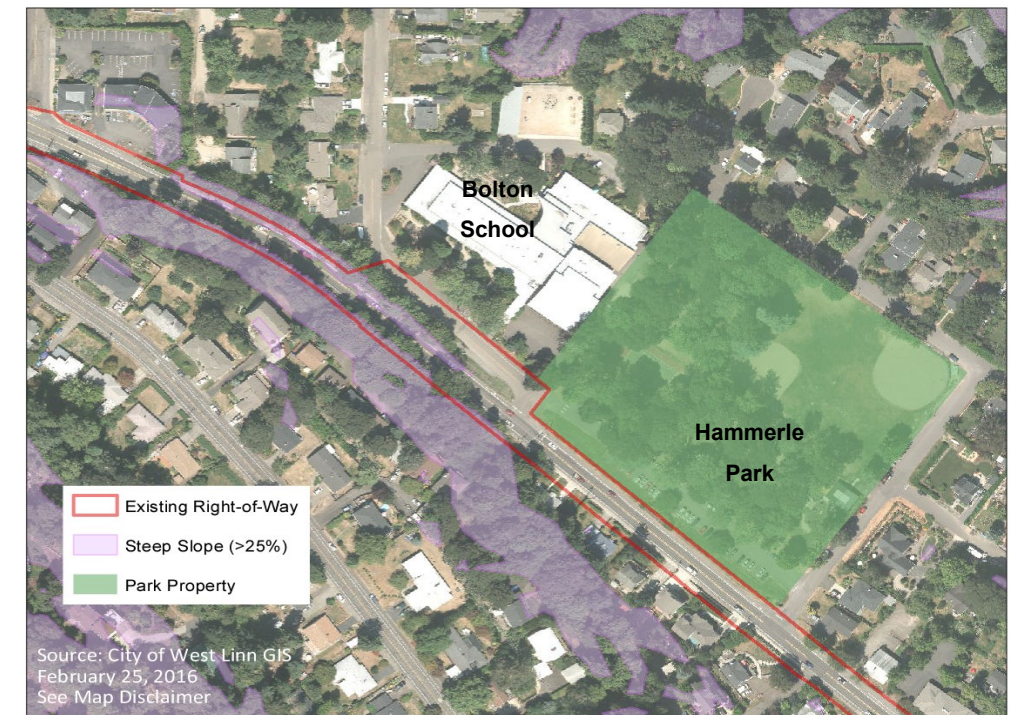
Varying right of way and steep slopes present challenges to the improvement of OR 43
