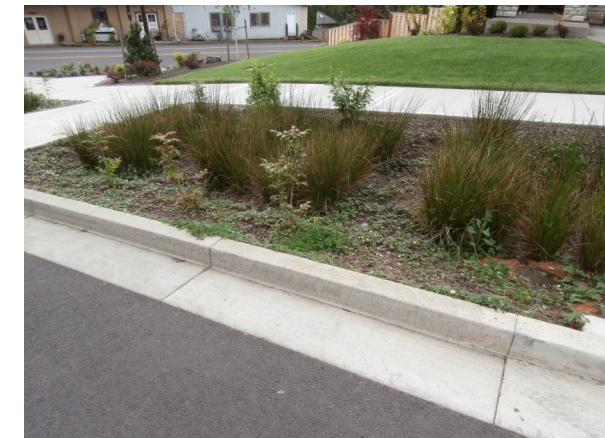
Example of rain garden Stormwater facility
