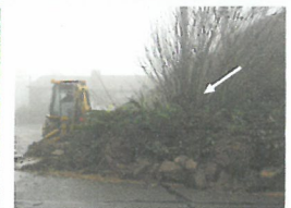
earth flow (unchanneled flow)
