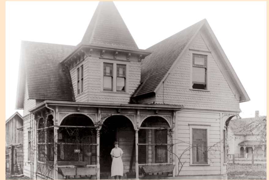
The Joseph H. Ralston House, ca 1910. See No. 30 on the tour.
