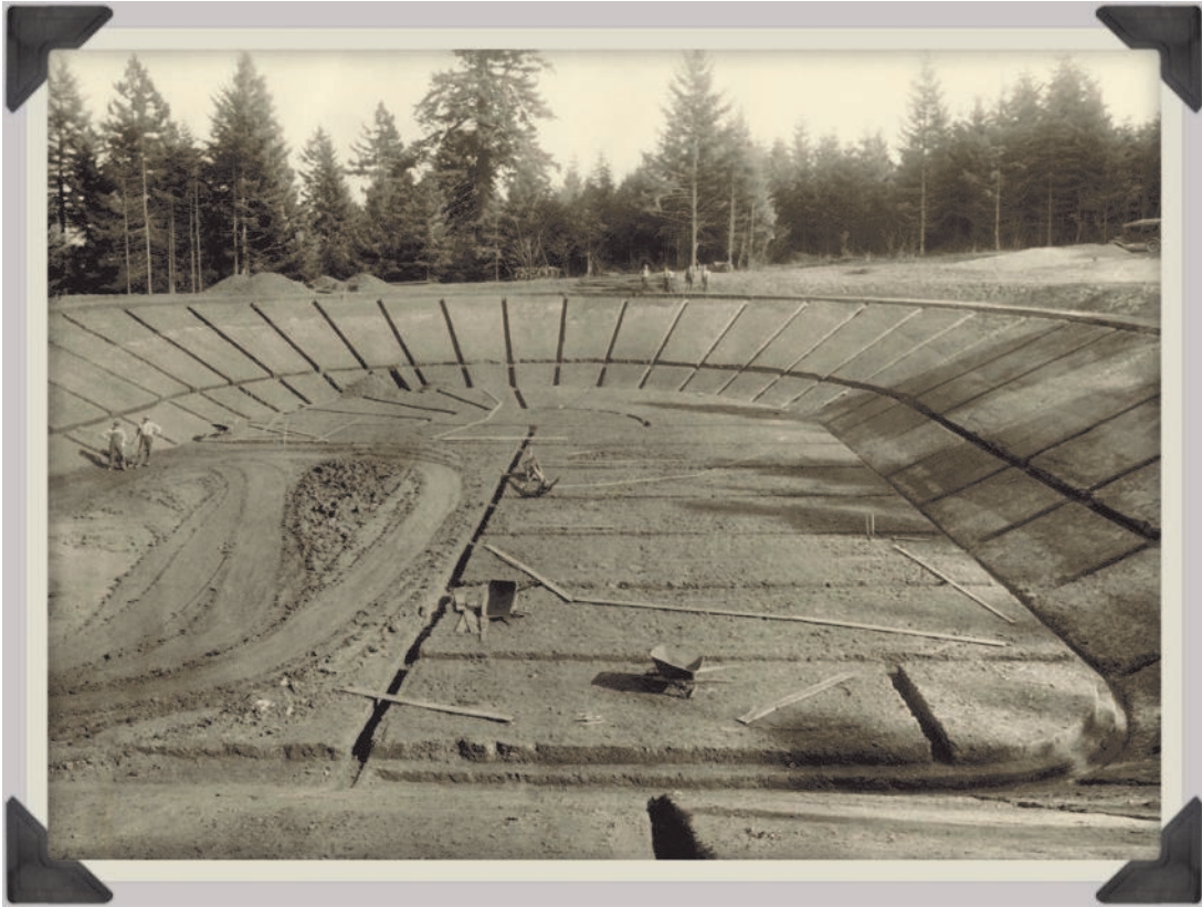
The 1913 Building of Bolton Reservoir
