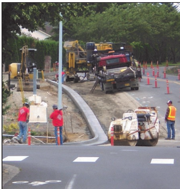
Widening of Santa Anita Dr. at Rosemont Rd. Traffic signal installation is planned at this intersection in the CIP as a TSP Action Plan Project.
